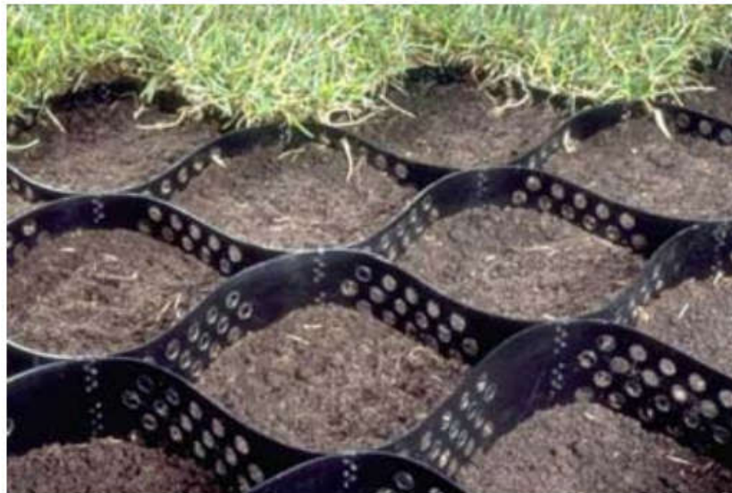
Figure: Geocells deployed for Slope Face protection application
